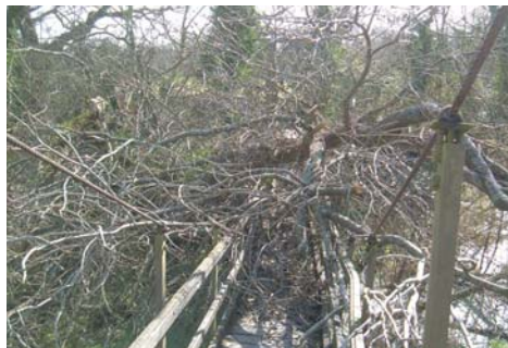
Fallen tree across the suspension bridge at North Stoke.
