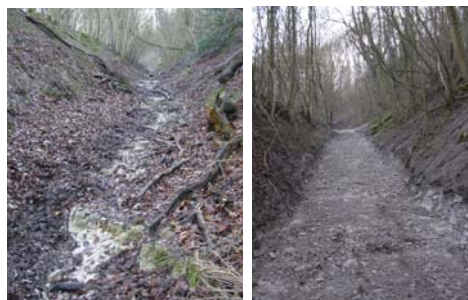
Re-grading of Telegraph Lane (Harting 884) - Before & After.
